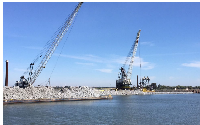
The State installed a salinity drought barrier to stop the encroachment of saline waters into the Sacramento-San Joaquin Delta due to the lack of freshwater flows.
