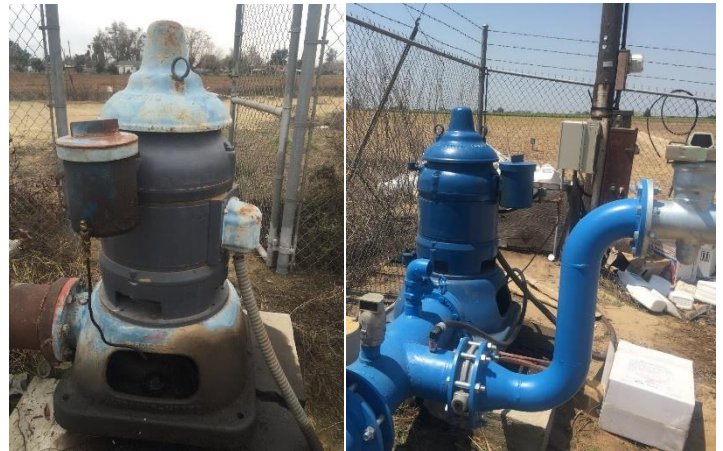
Figure 2. Turbine pump on a small-scale Southeast Asian farm, before and after improvements to increase energy efficiency funded by SWEET
