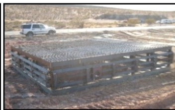
Photos before and after the AMLU helped to install a cupola over a 1,600-foot-deep abandoned mine next to Highway 395, Kern County.
